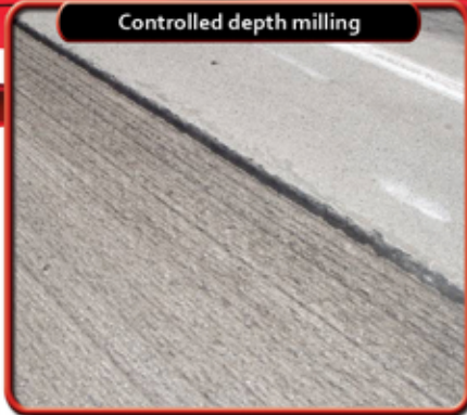
Controlled depth milling - RH4060 preparing turn lane for overlay
