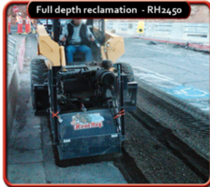
In place recycling - RH2450 mixing parking lot, materials to be reused as base
