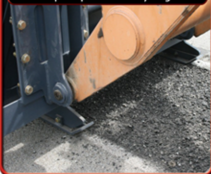
Two pass cut prior to utility installation
