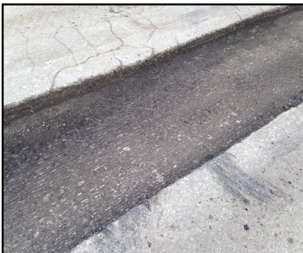
Milled edges provide an excellent bonding surface
