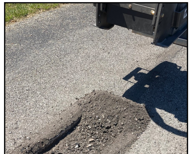
Cut material is suitable for reuse as backfill
